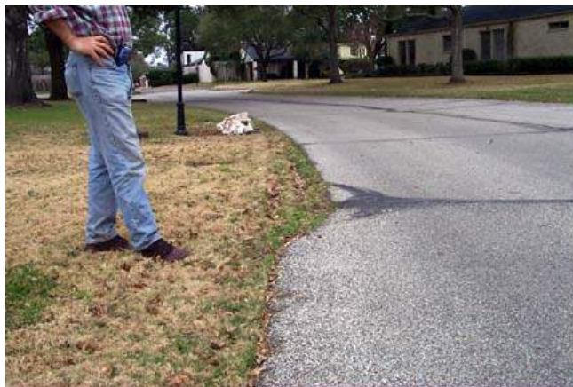
Figure 57 – GPR Profile 2: Quail Valley, Looking West Along the Profile (circa 2005)
